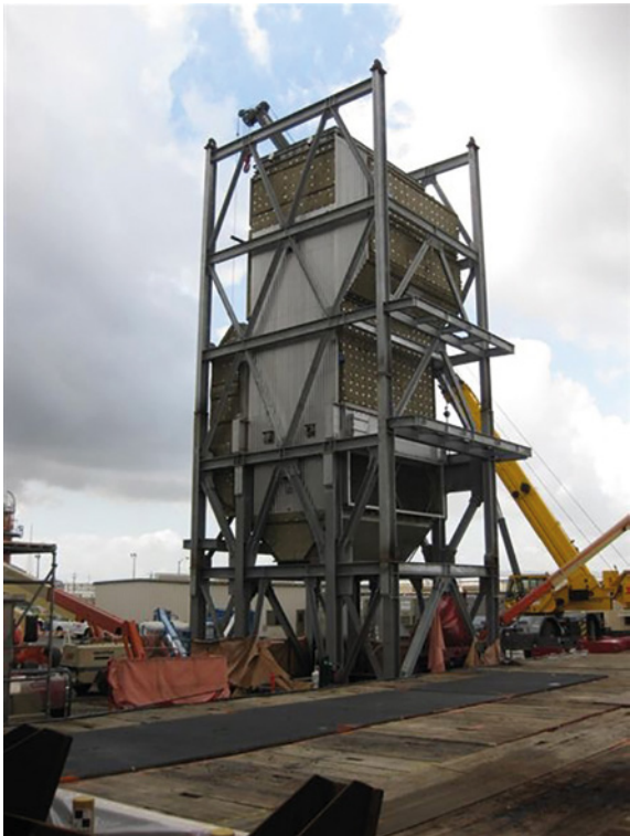
Figure 1. Heat Exchanger for combustion air preheating
